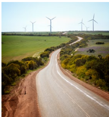
Walkaway Wind Farm in remote Western Australia.
